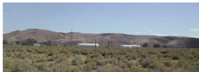
Storage Tanks near the Carlin Connection to UPRR
