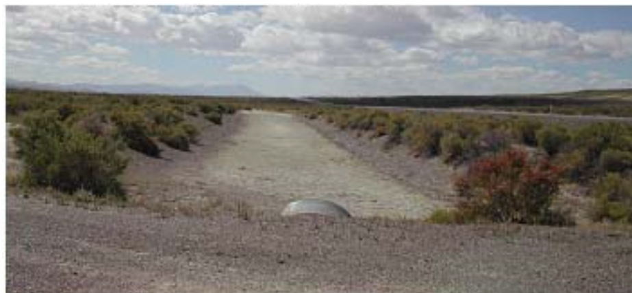
Culvert and drainage near S.R. 306
