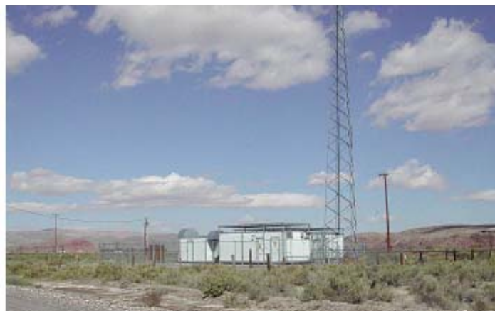
Tower near Carlin Connection to UPRR
