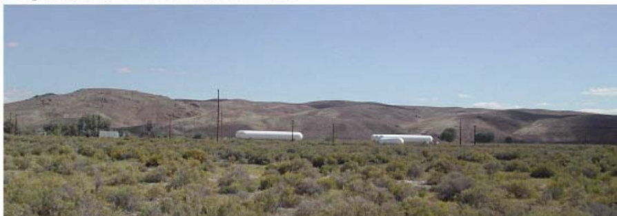
Storage Tanks near the Carlin Connection to UPRR
