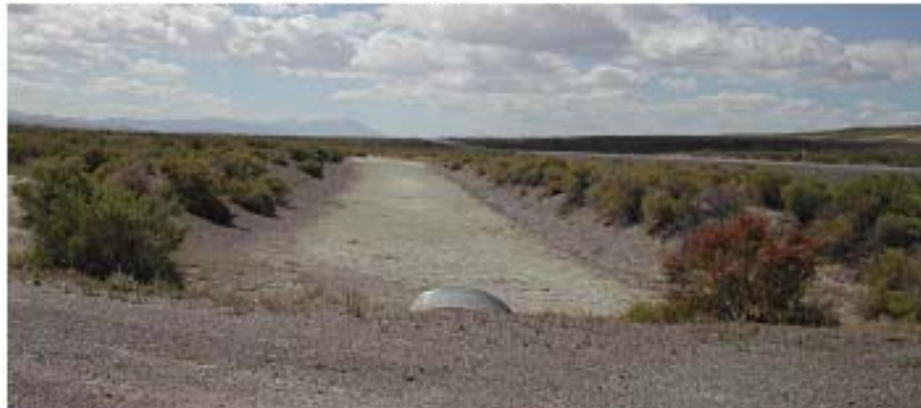
Culvert and drainage near S.R. 306
