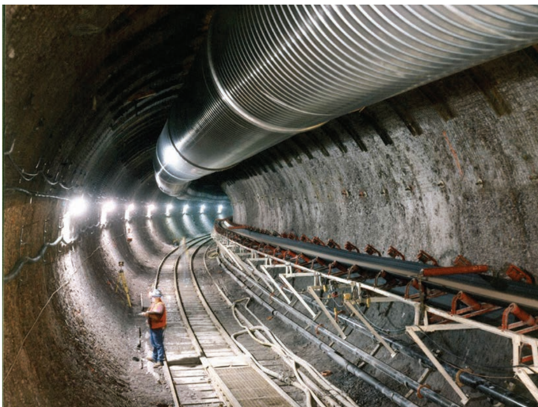
FIGURE 1.1. The underground Exploratory Studies Facility built at Yucca Mountain by the Department of Energy to determine whether the location was suitable as a deep geological repository.
